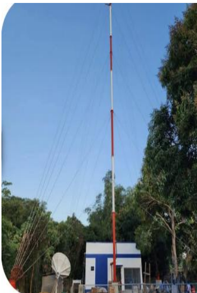
SITE LOCATION WITH TVRO
