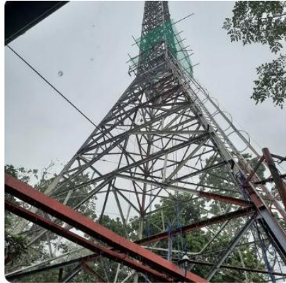
SITE LOCATION WITH TVRO
